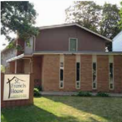
The current St. Francis House was formerly a convent. Built in 1956 for 12 sisters, it now houses 22 men and 30 women.
